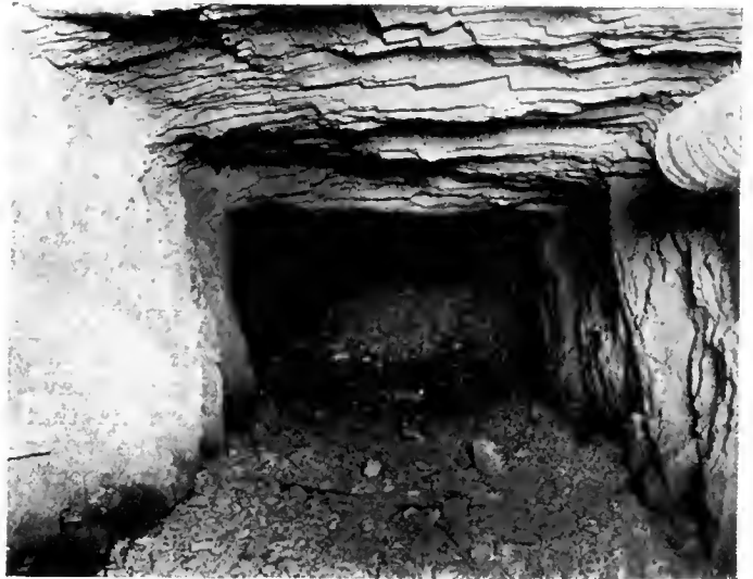
Final connection of the Pioneer Tunnel—Looking west
